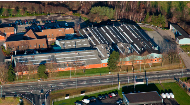
scansteel foodtech headquarters Site 1 - 10,450 m 2
